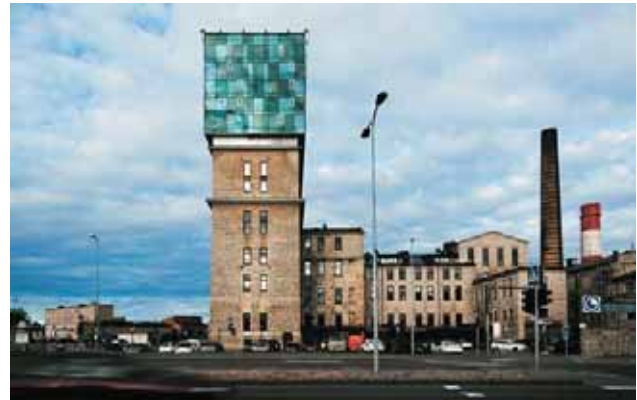
Figure-7: Integration of Limestone Wall and Glass. Source: https://www.kaidohaagen.com/photo_17316879.html
