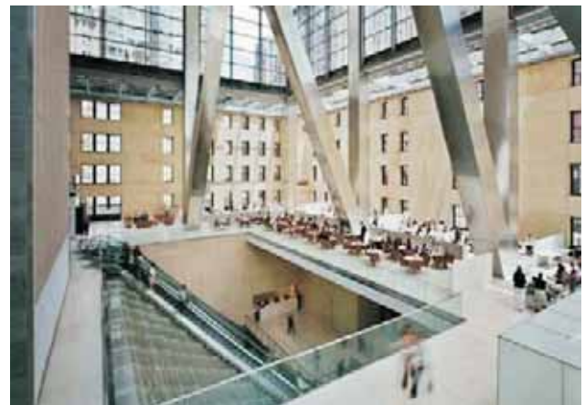
Figure-5: Use of Steel in Hearst Tower. Source: https://www.fosterandpartners.com/projects/hearst-headquarters
