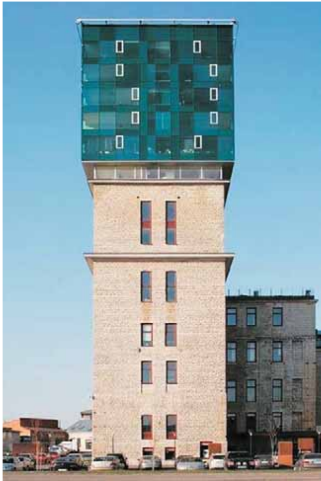
Figure-6: Integration of Limestone Wall and Glass. Source: https://www.kaidohaagen.com/photo_17316879.html
