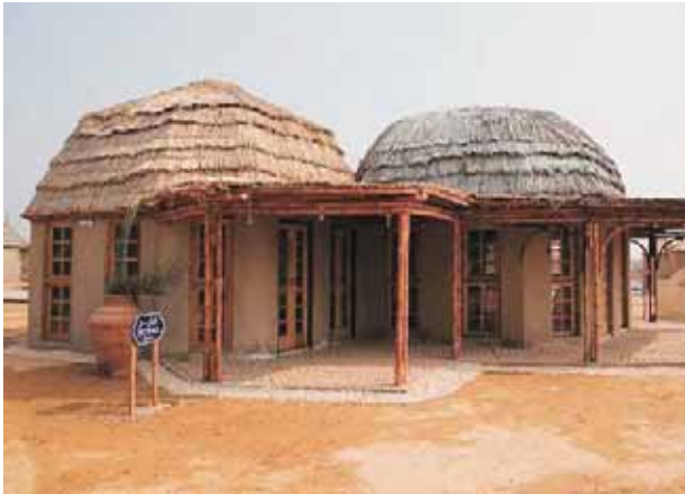
Figure-2: Usage of domed thatched rooftops and bamboo bracings for enabling thermal comfort and structural support as a part of the vernacular building tradition. Source: INTBAU 2019
