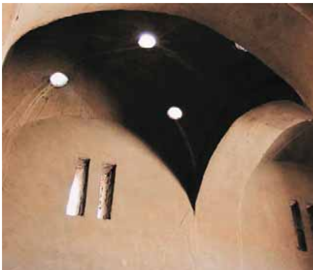
Figure-6a: Mud domes with smaller sized apertures ensure a more pressurized wind stream. Source: Laylin, 2010
