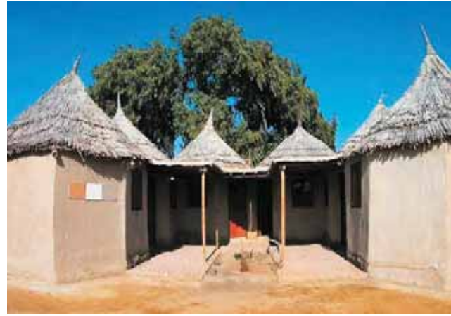
Figure-3: Usage of conical thatched rooftops for enabling thermal comfort as a part of the vernacular building tradition paired with mud plaster construction. Source: Lari, 2015
