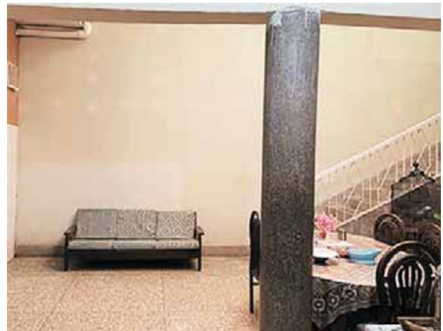
Figure-4: Terrazzo Wrapped up on Columns.
