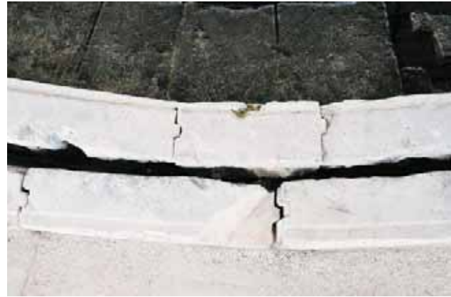
Figure-13: Coral construction tongue and groove joints, water tank in Fenfushi. Source: P. Pradines
