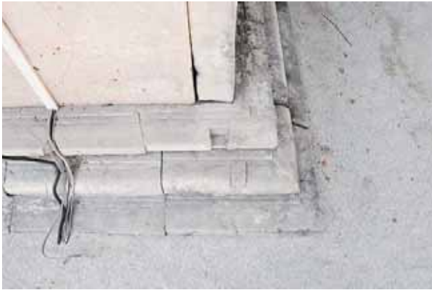
Figure-12: Coral construction dovetail joints and lap joints (zig zag), Meedhoo island raa Atoll. Source: S. Pradines
