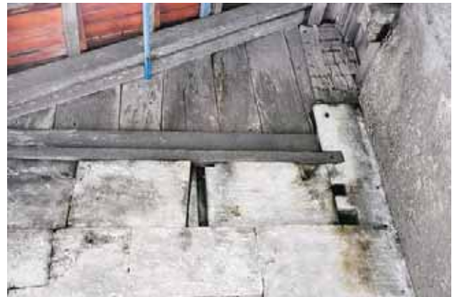
Figure-11: Coral stone buildings without mortar and wood techniques with peg holes, Meedhoo island raa Atoll. Source: S. Pradines
