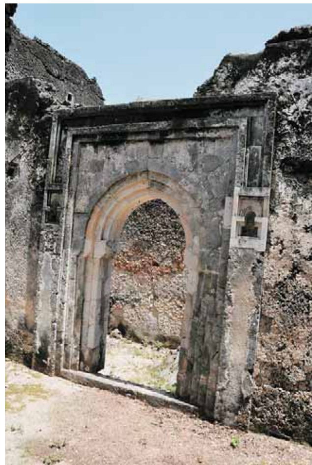
Figure-9: Fresh marine coral door frame in the palace of Songo Mnara a 15th century Swahili site. Source: Pradines
