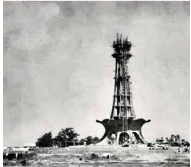
Figure-6: Construction of Minar-e-Pakistan Source: Khan, 2015
