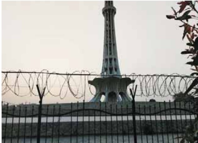
Figure-8: Fence around the National Monument
