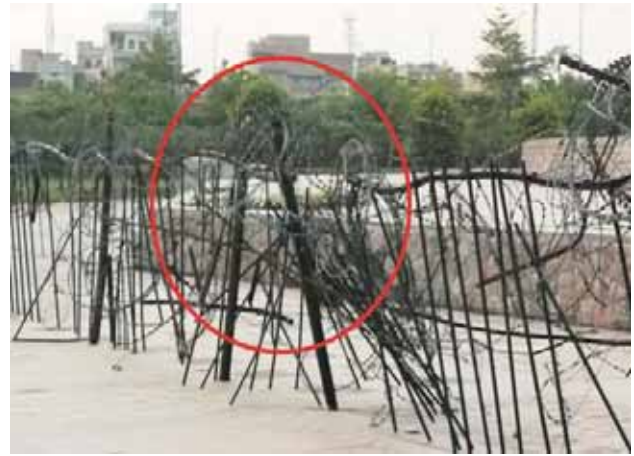
Figure-9: Entrance toward the National Monument
