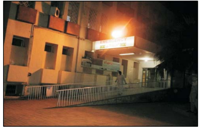
Figure-8: Lack of Shade and Poor Lighting on the Main Access of the A&E Department.
