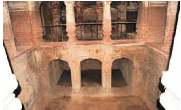
Figure 14: View of Basement and Sub-Basement
