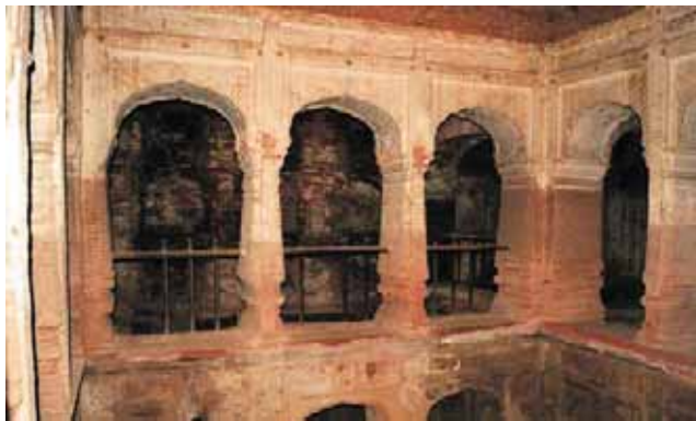
Figure 13: View of Basement Showing Typical Sikh Style of Architecture
