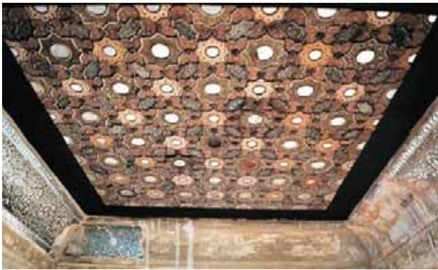
Figure 9: Interior View of Ceiling Stucco Work with Decorated Concave Mirror
