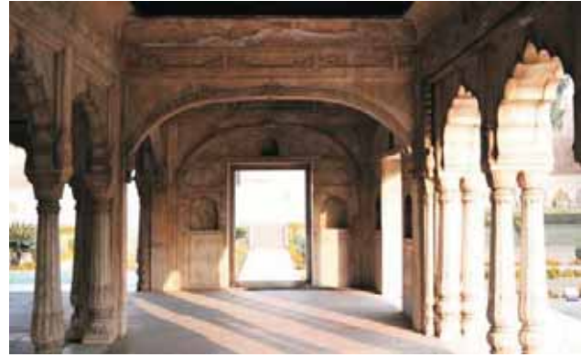
Figure 8: Interior View of Ground Floor
