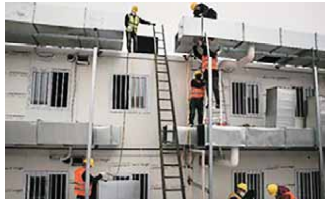
Figure-5: Designated Services Ducts for HVAC & Plumbing. Source: Wuhan, 2020
