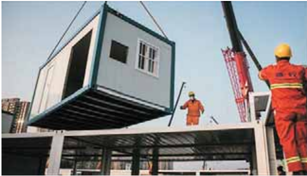
Figure-2: Prefabricated / Portacabin Units During Construction. (Source: Wuhan, 2020)
