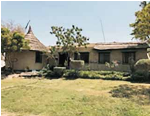
Figure-18: Exterior View of Visitor's Center
