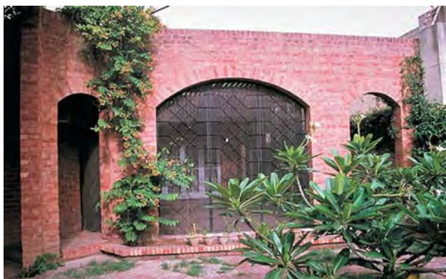
Figure-3: Wall Creepers Covering Exterior Facade. Source: www.googleimages.com
