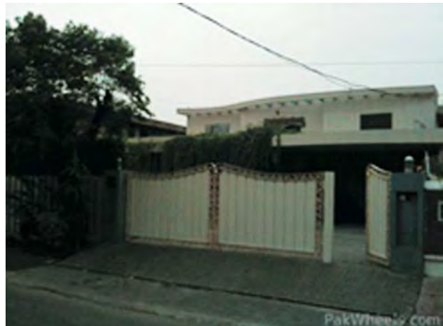
Figure-10: Front View of Modern House.
