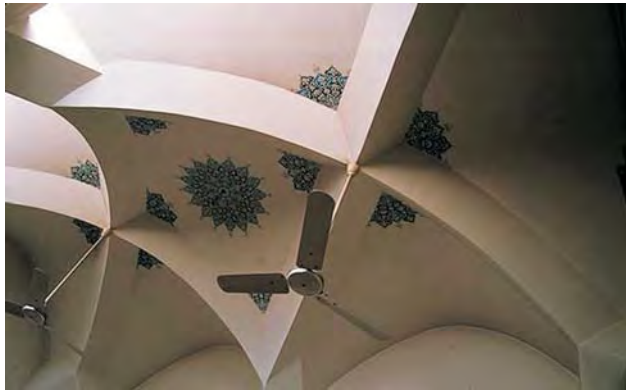
Figure-5: Vault structure and floral patterns on ceiling. Source: www.googleimages.com
