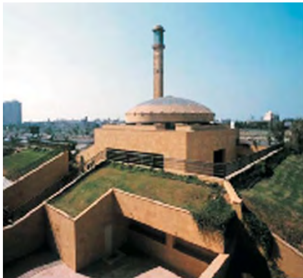
Figure-3: Monumentality in architecture. Source: Info 360, 2017
