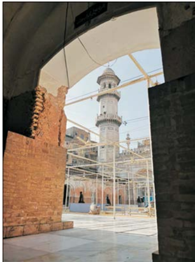
Figure-2: Proportions of elements portray a feeling of stability and amity- broad and massive looking towers.
