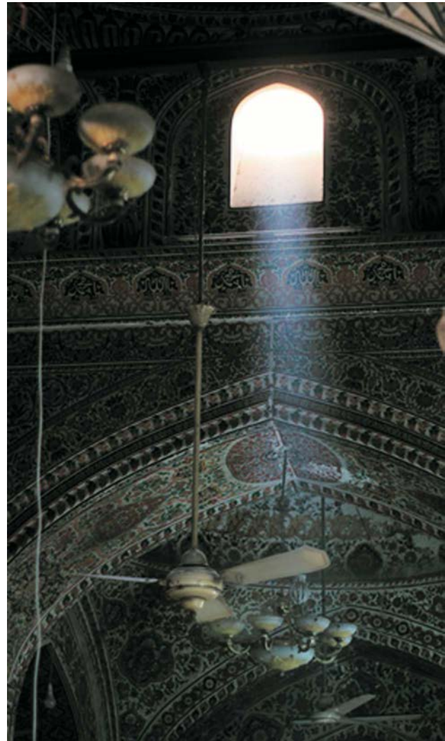
Figure-14: Detail-small niches given at the base of the domes to allow natural sunlight to illuminate the west side walls of the mosque.
