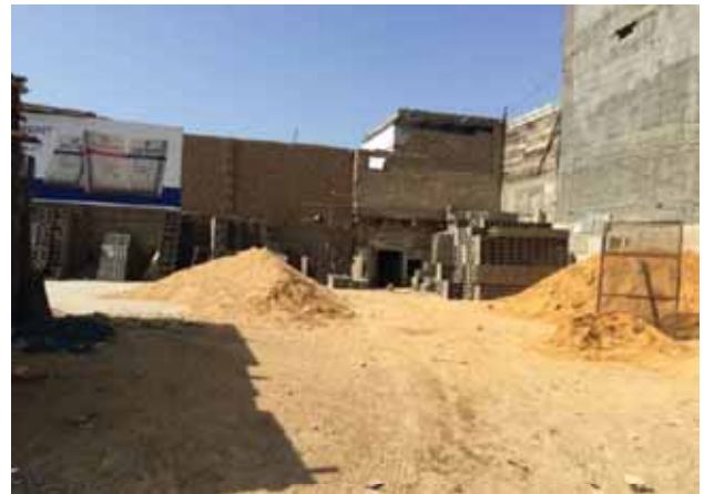
Figures 10: Another construction yard at Machar Colony
