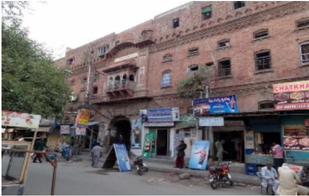
Figure 2: Front Façade of DAV Hostels Source: Islam, Mustafa and Kabir, 2016
