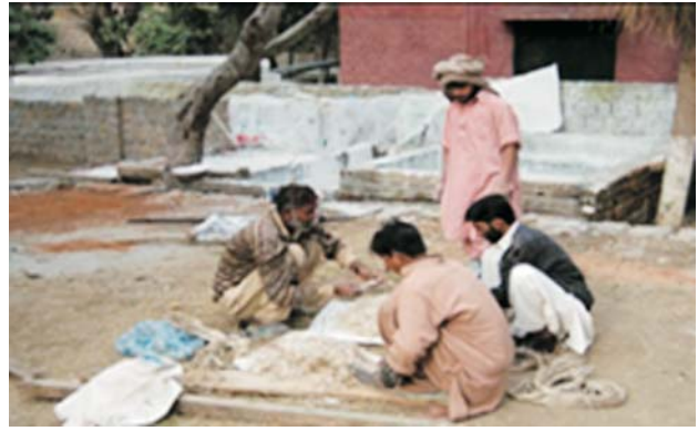
Figure 11: Preparation of Mughal lime plaster on site with traditional methods.
