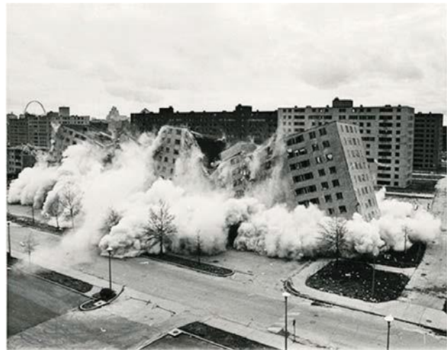
Figure 1: The demolition of Pruitt-Igoe in 1972 fueled resistance to deterministic thinking (Golembiewski, 2014).
