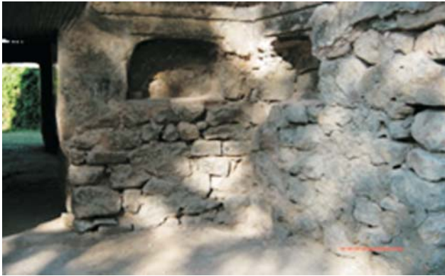
Figure 10: Interior views before conservation works.
