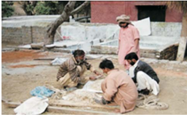
Figure 11: Preparation of Mughal lime plaster on site with traditional methods.
