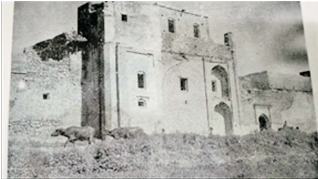
Figure 15: View of main gate of Shahjehani Sarai vanished from the scene due to illegal occupation (Siddique, 1977).
