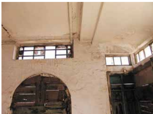
Figure-28: Dampness on walls seen in the interior.
