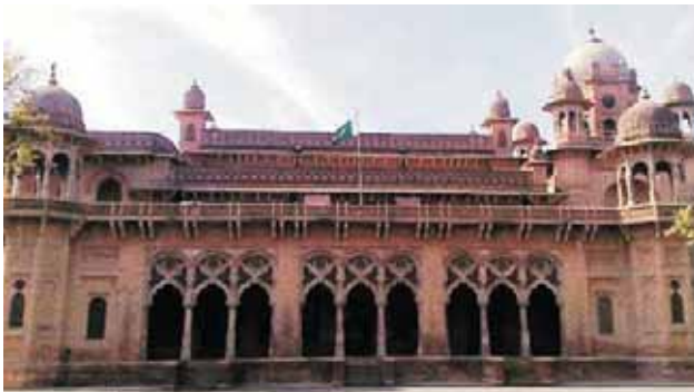
Figure-2: The elevation of old building of Aitchison College Lahore.
