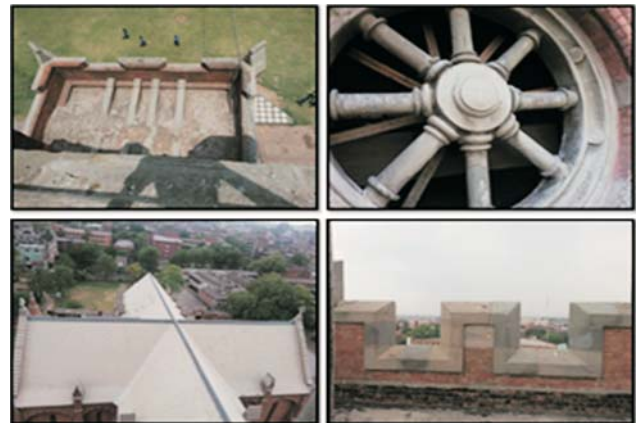
Figure-14: Different views of roof top.
