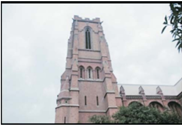
Figure-17: View of the Tower reaching great heights including gothic details of pointed arches, buttresses, trefoil openings, and sloping roof at the rear.
