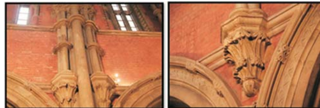
Figure-9: Decorative Collonettes on the Walls around the Nave.
