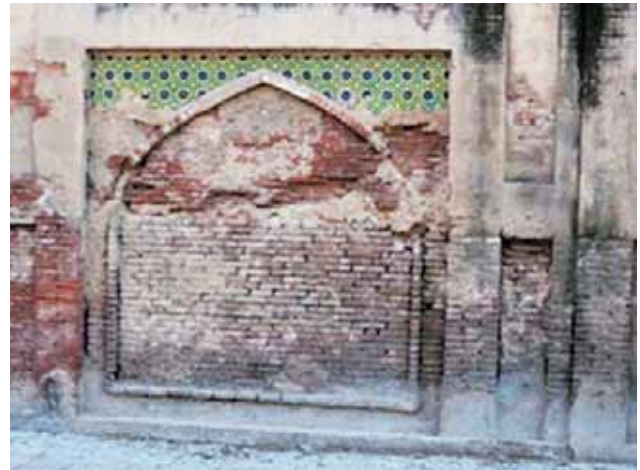
Figure-6: Defective plaster rendering of Shish Mahal
