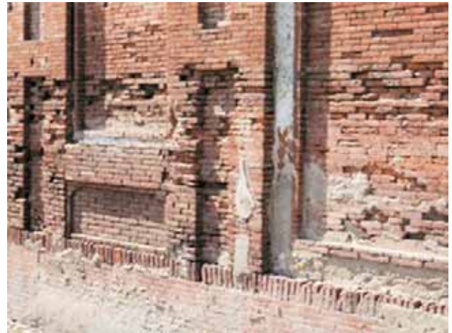
Figure-1: Deteriorated bricks.
