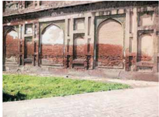
Figure-3: Dampness on brick wall.
