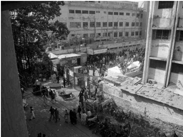
Figure-8: Civil Hospital Emergency center entrance.
