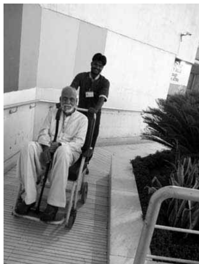
Figure-1: Ziauddin Hospital Clifton Karachi: Entrance Ramp does not have a hand rail.
