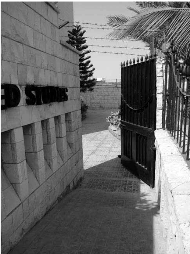
Figures-9, 10: Entrance of a local school, showing a ramp and steps for accessibility to classrooms.
