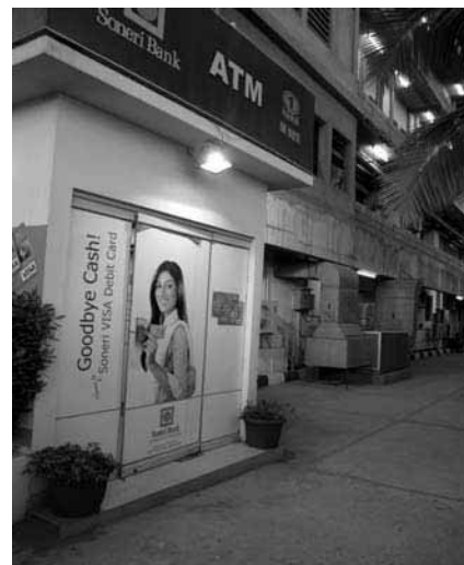
Figure-2: Ziauddin Hospital Clifton Karachi: ATM room un-accessible to people with disabilities.
