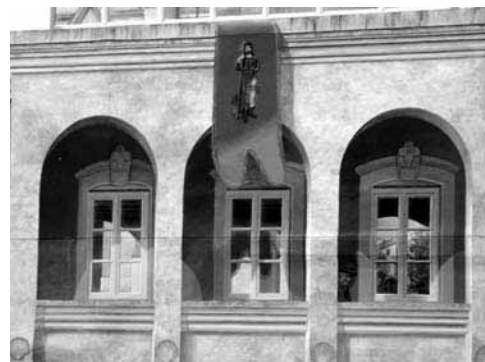
Figure-11: Public art used to animate a restored blank façade, Montpellier France.
