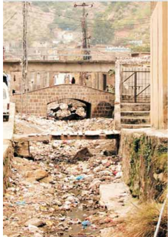
Figure-29: The nalla is filled with garbage between houses
