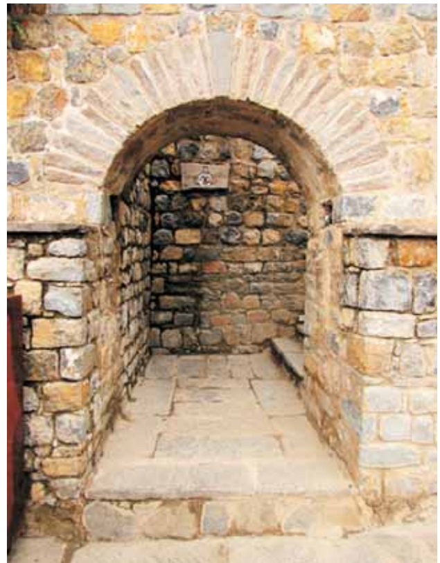
Figure 12: Doorway and steps leading to hotspot on hillside
