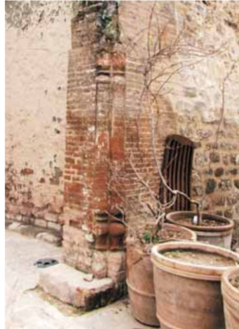
Figure-33: Remnant of old decorative brick columns
