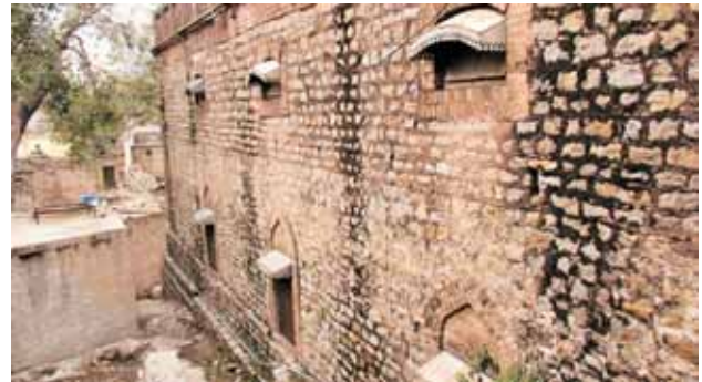
Figure-30: The back facade of the dharamshala
