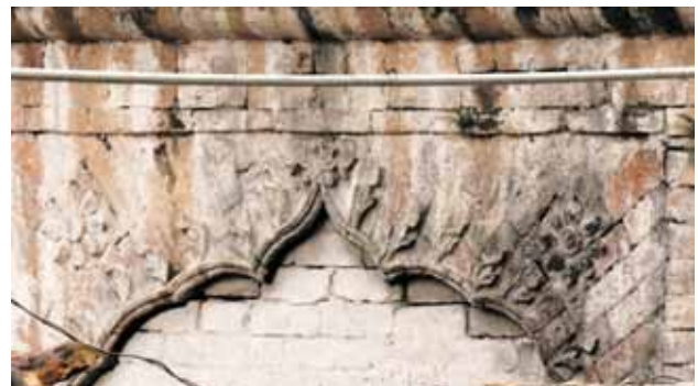
Figure-31: Decorative brick work on a doorway
