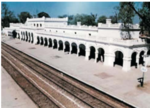
Plate-11: Railway Station
