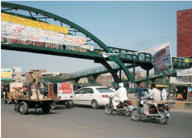
Plate-12: Overhead Bridge by HMC, Taxila
