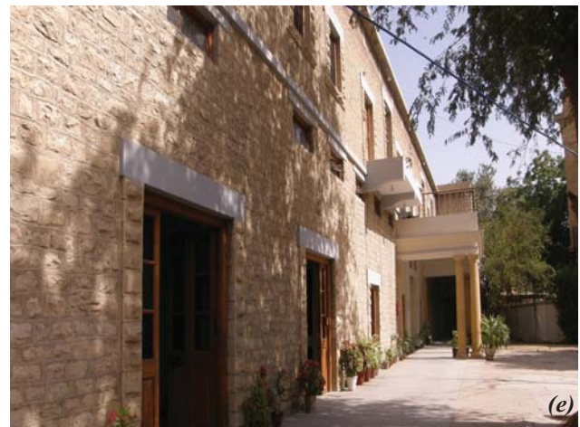
Figure-6(a-e): The entrance portal in building #1. (a) Entrance portal embedded inside later additions. (b) Removal of later additions. (c) The carved out entrance portal. (d) At the stages of repairs and re-cast slab. (e) The restored entrance portal at completion of works.
