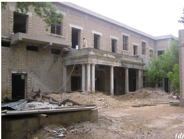
Figure-6(a-e): The entrance portal in building #1. (a) Entrance portal embedded inside later additions. (b) Removal of later additions. (c) The carved out entrance portal. (d) At the stages of repairs and re-cast slab. (e) The restored entrance portal at completion of works.
