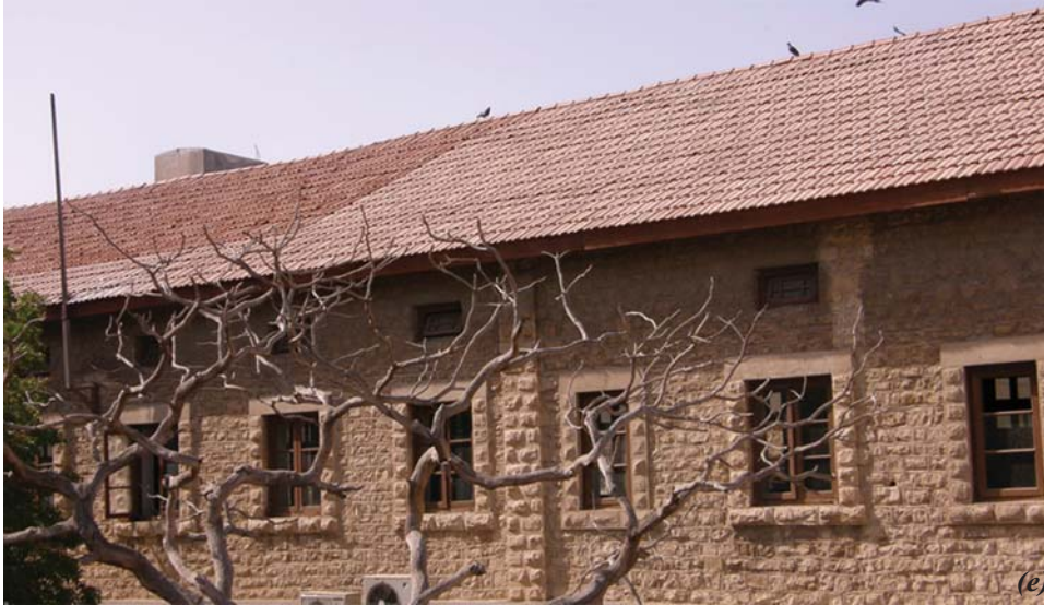
Figure-7(a-e): The original timber pitched roof spanning over a large hall on first floor of Seth Fatechchand Khilwani Block (building #2) was in a highly dilapidated condition with most of its purlins infected with termite. Only the completely destroyed timber was replaced whereas all the original trusses were cleaned and treated with protective timber coating. The terracotta tiles were also re-used; only the damaged ones being replaced. Since the complete restoration of this space as an 'exhibition and display hall' is still on hold due to lack of funds it is becoming more and more difficult to keep the restored roof in a maintained condition.
