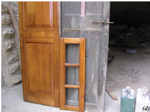
Figure-5(a-e): Cleaning and polishing of timber works. (a) Tagging and numbering of door/ window shutters. (b) Application of solution to soften existing paint layers. (c) Scrapping of paint layers and smoothing of timber surfaces. (d) Polished finish of cleaned timber elements. (e) Final finished door panel.
