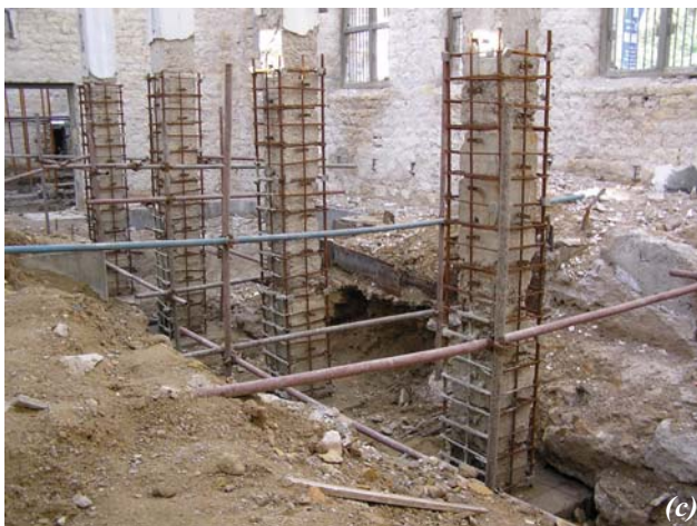
Figure-3(a-d): The restoration process cycle; (a) Deteriorated bases of the RCC column. (b) Temporary propping for relief of loads and chipping/ surface preparation of beams. (c) Reinforcement details for strengthening of lower half of columns. (d) The columns after jacketing; at curing stage.
