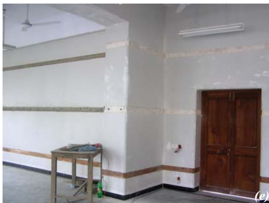
Figure-4(a-f): Lime plaster of stone masonry walls. (a) Removal of existing damaged lime-plaster. (b) Stone masonry walls as exposed after complete removal of existing plaster. (c) Making lime-plaster. (d) Applying the new lime-plaster. (e) Masonry walls before complete finishing of plaster surfaces. (f) Masonry walls after complete finishing of plaster surfaces.
