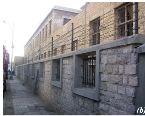
Figure-8(a-b): Restoration works along the Burns Road boundary wall involved demolition of RCC slabs built along the space between the building and the wall. These spaces had been in disuse for many years and became a hideout for drug edicts; a menace now removed from the vicinity due to clearing of area and restoration of the wall.
