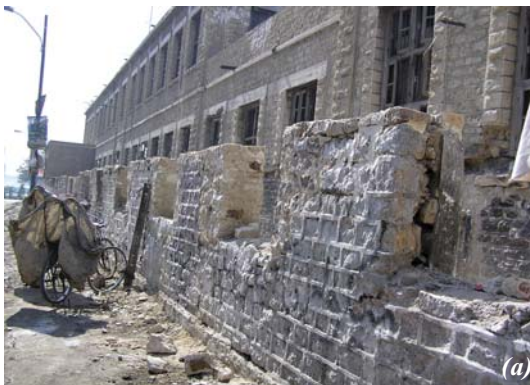
Figure-8(a-b): Restoration works along the Burns Road boundary wall involved demolition of RCC slabs built along the space between the building and the wall. These spaces had been in disuse for many years and became a hideout for drug edicts; a menace now removed from the vicinity due to clearing of area and restoration of the wall.
