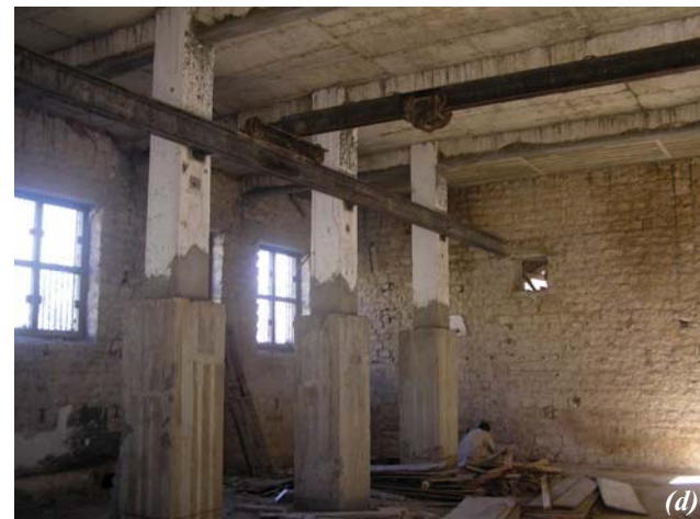
Figure-3(a-d): The restoration process cycle; (a) Deteriorated bases of the RCC column. (b) Temporary propping for relief of loads and chipping/ surface preparation of beams. (c) Reinforcement details for strengthening of lower half of columns. (d) The columns after jacketing; at curing stage.
