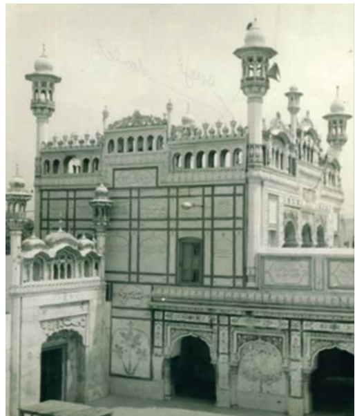
Figure-9: Mosque Abu al-Khair Nau Lakh Hazari Shahkot demolished in 2008
