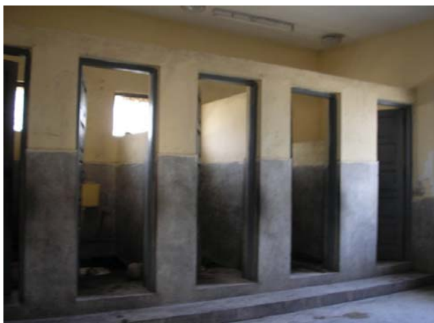
Figure-8: Inadequate washroom facility in F.G. JMS F-I-8/1.
