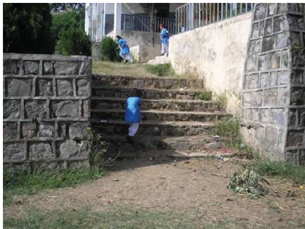
Figure-12: Unsafe stairs towards the play area F.G. JMS G-9/2.
