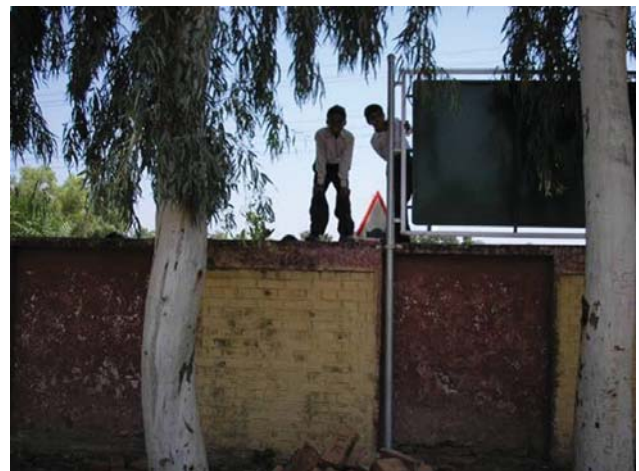
Figure-13: Insufficient height of boundary walls in F.G. JMS F-8/2 and F.G. JMS I-8/1.
