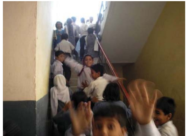
Figure-11: Insufficient width of staircase in F.G. JMS I-8/1.
