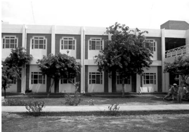
Civil Engineering, Department, Bahauddin Zakariya University (BZU), Mutlan.
