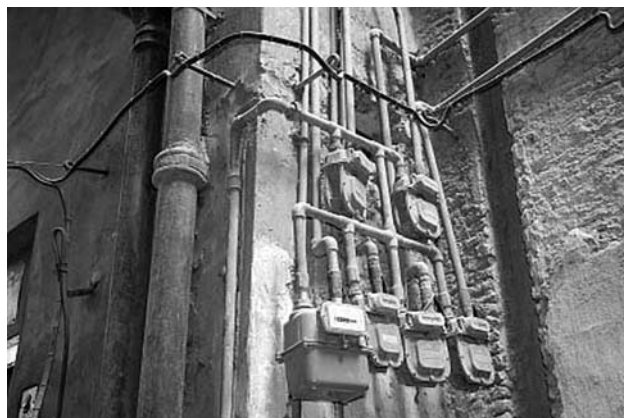
Figure-9: Meters for Sui Gas Supply Lines.
