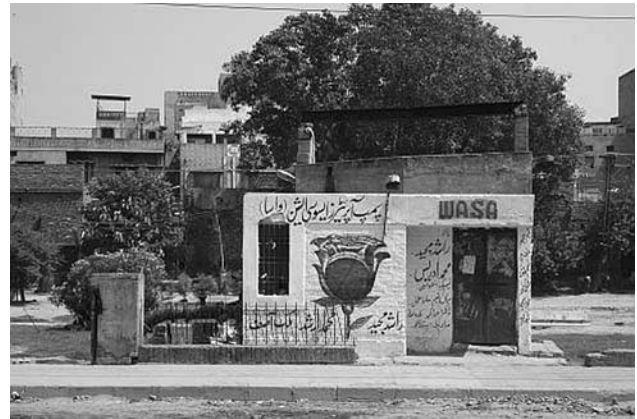
Figure-3: Tube Well located in Circular Garden.
