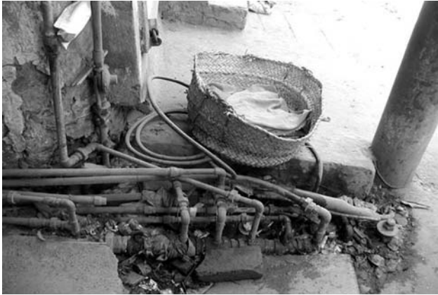
Figure-4: Water Supply Connections in Street.
