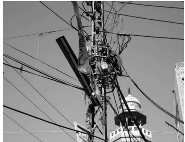
Figure-7: Transformer and Electricity Services near Masjid Wazir Khan.
