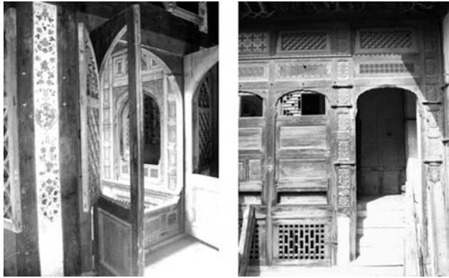
Figure-6 & 7: (L) Ground floor SW balakhana. (R) First floor dalan.
