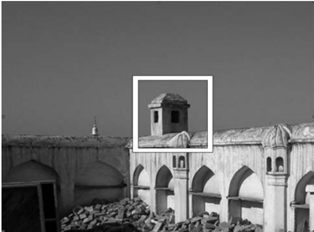
Figure-17: The chimney of the ventilation duct on NE side.
