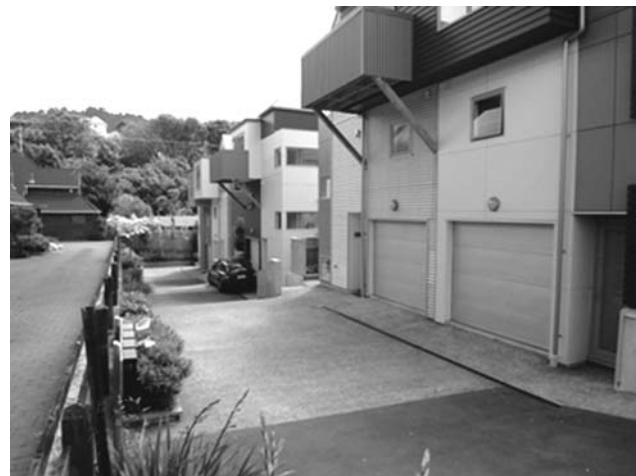
Figure-1: A recent five unit development in a suburban area of Wellington showing the dominance of paving to accommodate the motorcar.
