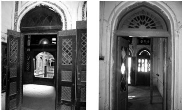
Figure-9 & 10: (L) Rooms open up to one another. (R) Circulation of air through open rooms.
