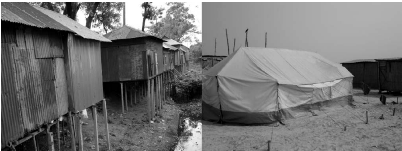
Figure-1: Inappropriate choice of building materials like C.I sheet & PVC sheeting.
