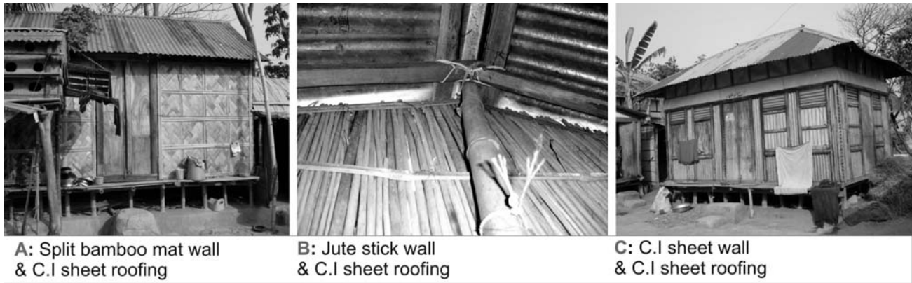
Figure-18: Three types of houses with their different walling material at homestead-01.
