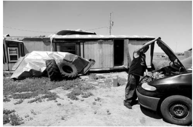
Figure-3: The Roma enclaves of Rome are just one variant on an old theme: the ethnic ghetto. Housing on the Pine Ridge native American reservation in South Dakota is similar in style, materials, and general disrepair. (photo: Kristina Barker for the Rapid City Journal)
