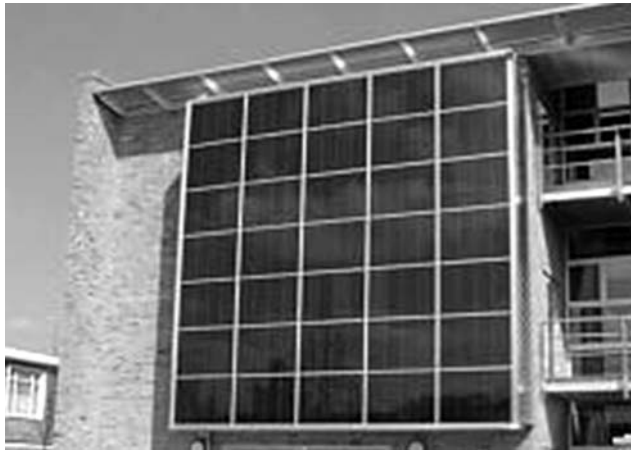
Figure 8: The South facing photovoltaic facade. Source for Fig 3 to 8: The Environmental Building: A Model for the 21st Century, manual by BREEAM).
