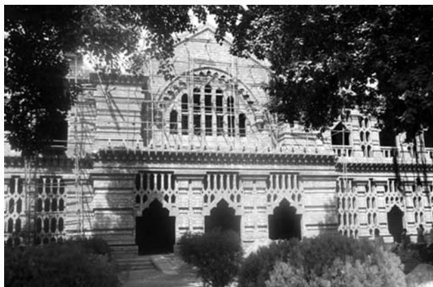
Figure 1: Eastern Elevation of Newly Constructed W.W. of LHC Building
