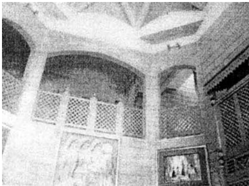
Figure 26 - 29: Azra Shaheen House, Khayaban-e-Hilal, Phase-VI, DHA, Karachi, finished in 1998. Organized around a central atrium. Fig 28 & 29 the house uses fair-faced load-bearing concrete block walls and pyramidal domes supported by concrete beams. Photos by Hassan Abbasi, 3rd Year, Dept. of Architecture, NED.
