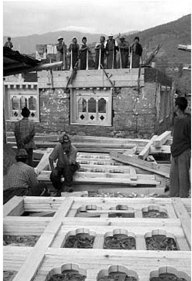
Fig-15: A house in Paro valley being reconstructed with the help of the community. The wooden windows are assembled on the ground before being held in place by the rammed earth. Professional carpenters or zopons build the rabse or timber framed walling and the women and men of the village help in building the rammed earth walling. (Lim, 1999)
