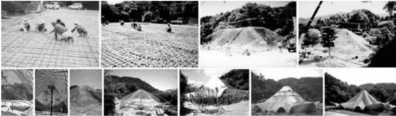
Fig-28: Building process showing the collaboration of local craftsmen in creating the bamboo woven interior ceiling. (Shoei Yoh website)
