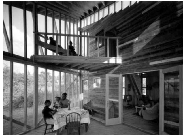
Fig-22: The ventilated porch opens up to the rest of the house. Costs for construction were kept down with the use of a tin roofing and recycled pine from an old church that was being razed nearby. (Hursely)
