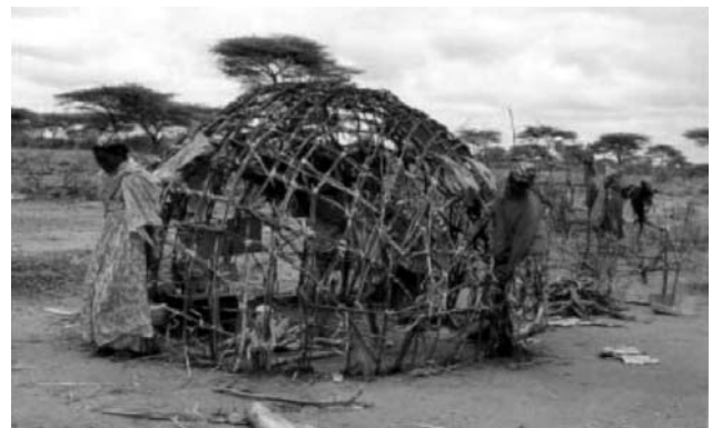
Fig-1: Constructing a Gabbra dwelling (Oliver 2003:30). It is the women that are in charge of constructing the dwellings. Lightweight and flexible poles from plant material are woven into a shell to be covered with fabric. The role of men would be to tend to the all-important source of livelihood which are the grazing animals.
