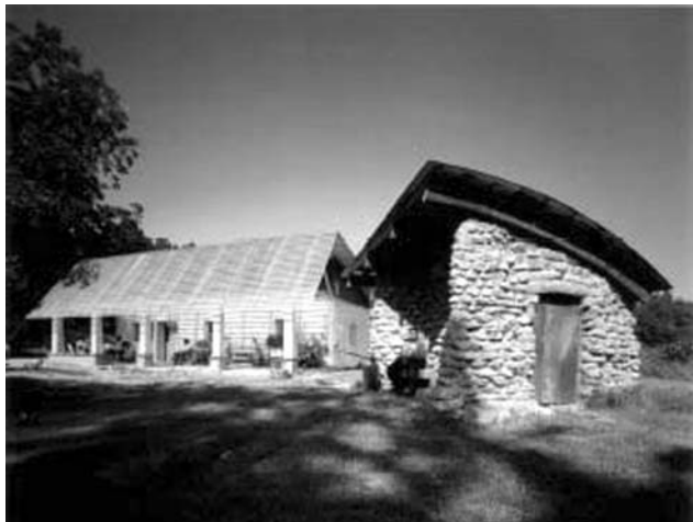
Fig-18: A separate structure was created as a smokehouse using discarded road signs for the roof and embedded glass bottles in the walls to admit light in and the walls of concrete rubble from a demolished silo. The main house features a porch reminiscent of local antebellum mansions. (Hursely)
