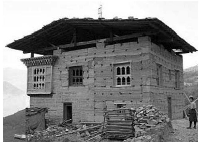
Fig-14: A newly constructed farmhouse in Paro valley built of rammed earth. (Lim, 1999)
