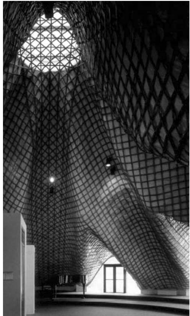
Fig-27: Construction process for this building involved the weaving of a bamboo grid by the local craftsmen which was suspended over the site and formed into the undulating shape which was then covered with a steel mesh and poured concrete. An important part of the process was the participation of the local craftsmen in the building process. The collaboration between the basket weavers, the architects, engineers and builders allowed for the development of an innovatively designed building.
