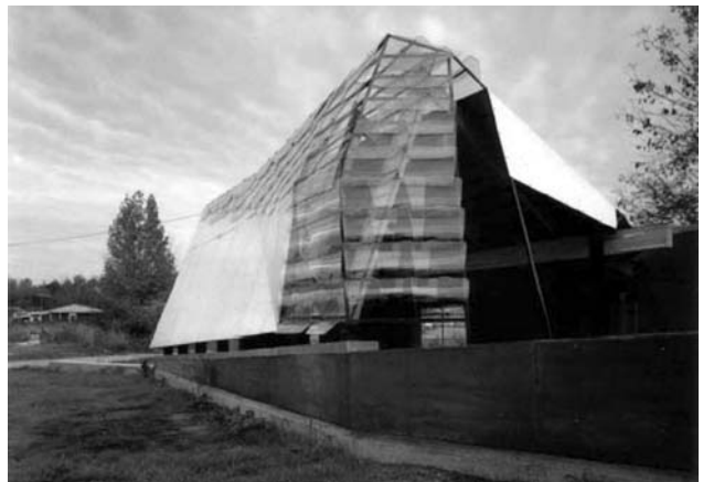
Fig-20: Mason's Bend Community Centre built in 2000 was constructed of rammed earth and recycled automobile windshields. The low, close to the ground form is in keeping with the community's vernacular forms and shapes. (Hursely)
