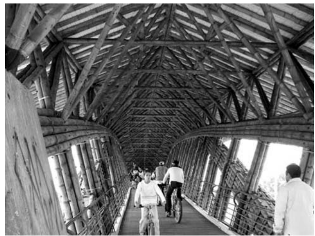
Fig-26: The Jenny Garzon Bridge in Bogota by Velez is a large scale hanging bridge capable of carrying the weight of pedestrians and cyclists. (Ajay Khanna)
