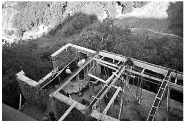
Fig-6: Working in partnership with European builders and partners, traditional building techniques were reinforced with new building methods such as the use of concrete and steel bars to stabilise what would have been mud and stone walls. (Kasbah du Toubkal website)
