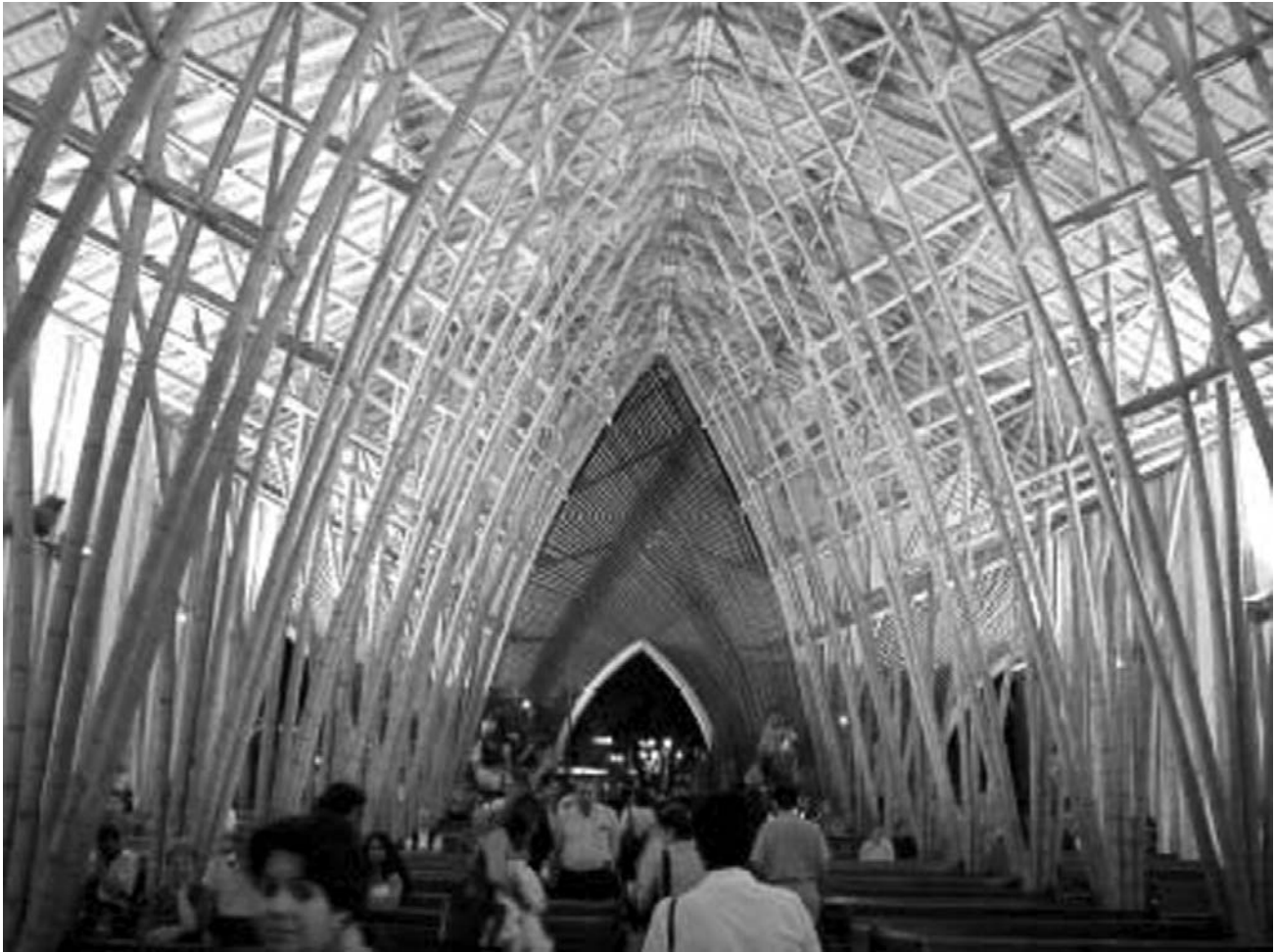
Fig-25: The Guadua Cathedral at Pereira, Colombia. The architect Simon Velez works with the specie of giant bamboo guadua creating large, structures by incorporating innovative joinery techniques. (Ajay Khanna)
