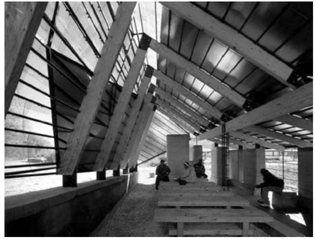
Fig-19: As in all of Rural Studio's projects, the community centre is a lesson in resourcefulness. The trusses and benches were created from laminated cypress donated by a studio supporter. The steel trusses were likewise a material donation. (Hursely)
