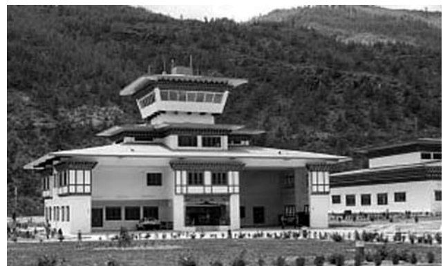
Fig-16: (all images on this page): The newly constructed Paro airport seeks to find a Bhutanese architectural identity by adopting architectural forms with historical precedents. The buildings are given a prestigious identity by the double jabzhi or double layered roof. The main structure is built of concrete but the windows and fenestrations use the traditional timber framing. Elaborate use of carved elements and paintings show the importance given to such a building which has become symbolic of the progressive changes that the country is undergoing. (Lim, 1999)
