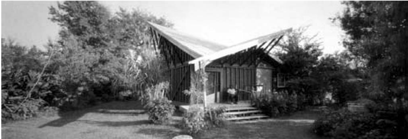
Fig-21: The Harris Butterfly House designed and built by Rural Studio architecture students in 1977. The steeply sloping roof, like butterfly wings were designed to channel rainwater to a cistern to be used for toilet and laundry and also to channel cool breezes into the house. (Hursely)
