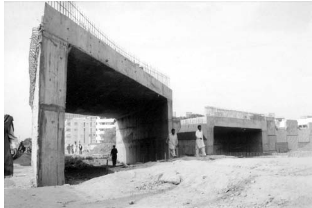
Figure 28 : The LEW under construction.
