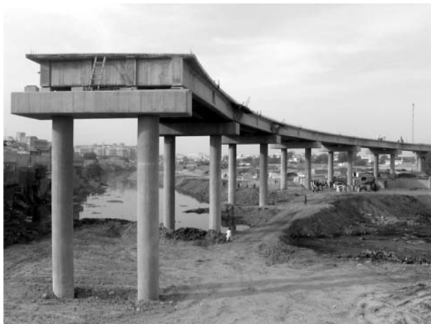
Figure 31: The LEW under construction at Sohrab Goth.
