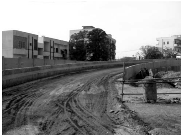
Figure 30 : The LEW under construction at Sohrab Goth.
