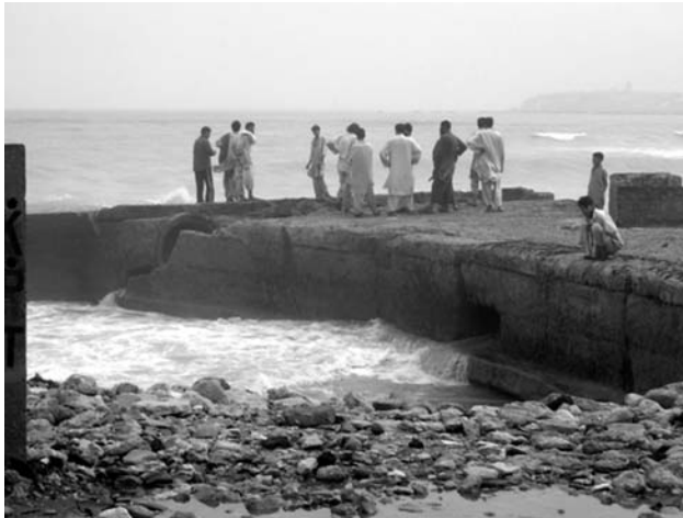
Figure 25 : Untreated Sewerage Disposal in the beach with in KPT Jurisdiction
