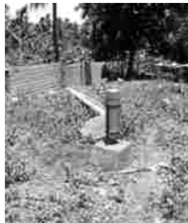
Figure 19: Quezon Rainfall Gauging Station - an example of community-based early warning system installed for threat prediction in flood prone areas in municipalities of REINA. Source: http://www.wmo.ch/web/homes/WWF4/Flash%20Floods/CountermeasuresDebrisFlow&Flashflood.pdf
