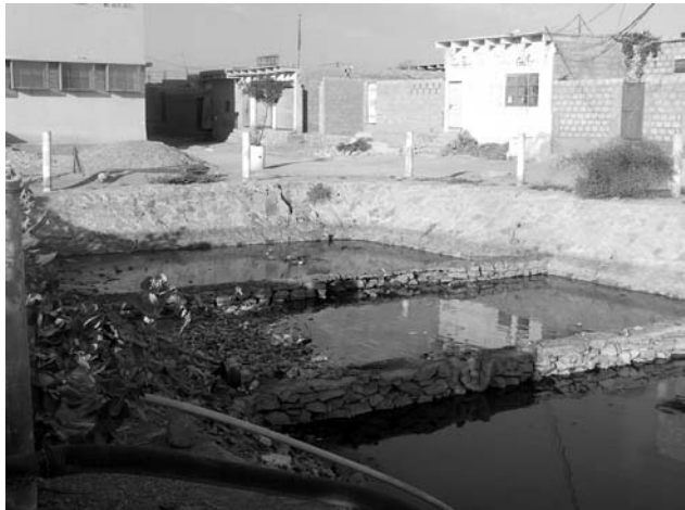
Figure 18 : Windmill with sewage treatment plant installed by Saiban.
