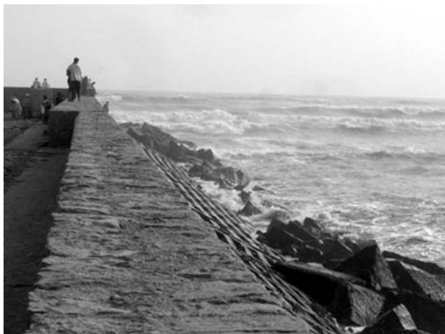
Figure 7: Walling at the beach are made with indefinite Engineering Standards of Construction.
