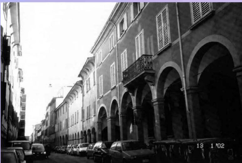
Typical Buildings after the Restoration. (Source: Dr. D. Binan Archives)
