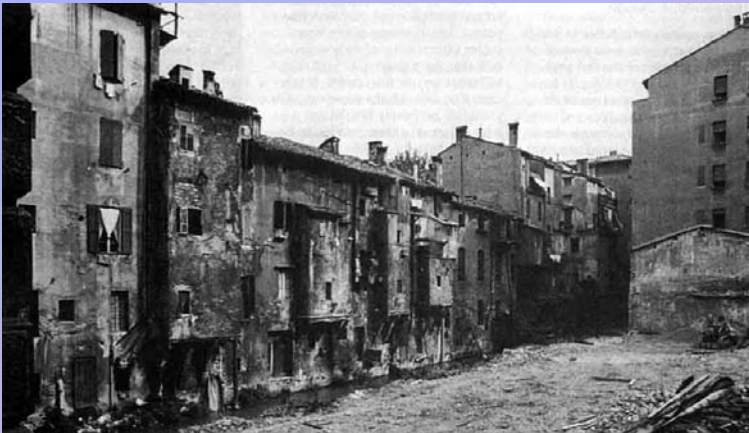
Deteriorated Conditions in the Historic Core Prior to the Beginning of Preservation Programme. (Source: Pier-Luigi Cervellati)
