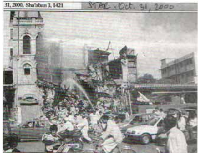
A pre-1947 building was completely gutted when it caught fire early this morning. At least 11 fire tenders were used to put out the fire in which 9 firemen were injured.—STAR photos Figure 6: A Historic Building that got Completely Destroyed by Fire within Three Hours.
