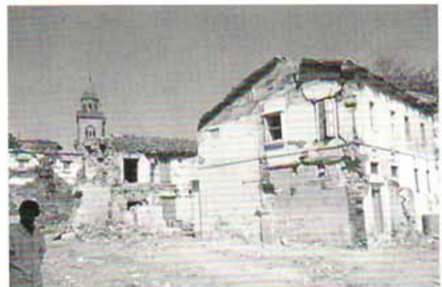
Figure 1: Historic Town of Bhuj Devastated by 2001 Gujarat Quake in India
