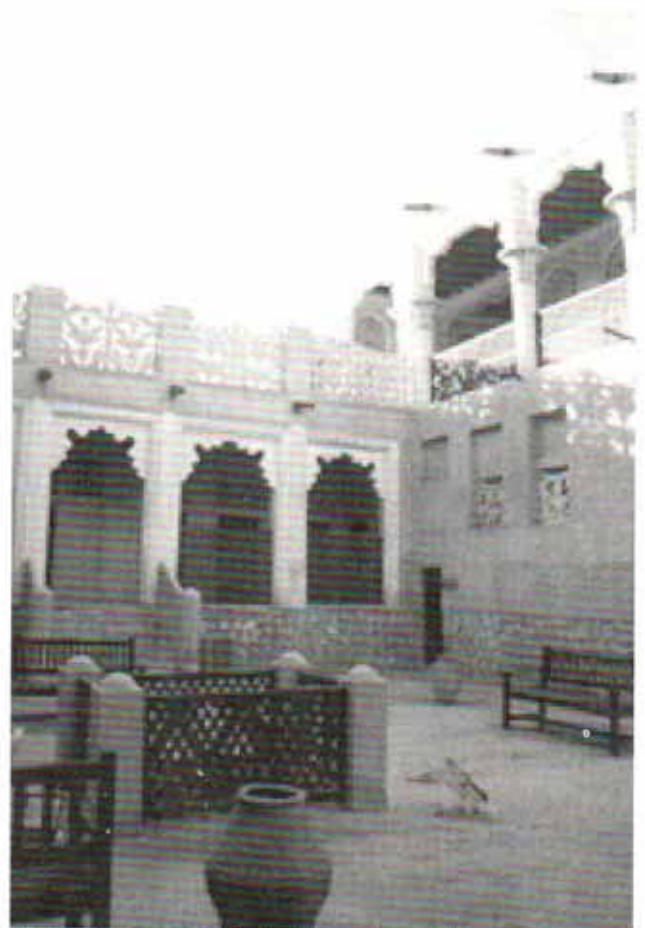
Figure 2: Specially Crafted Teak Doors, Plaster screens and Cornices used in reconstructed houses within Bastakia District.
